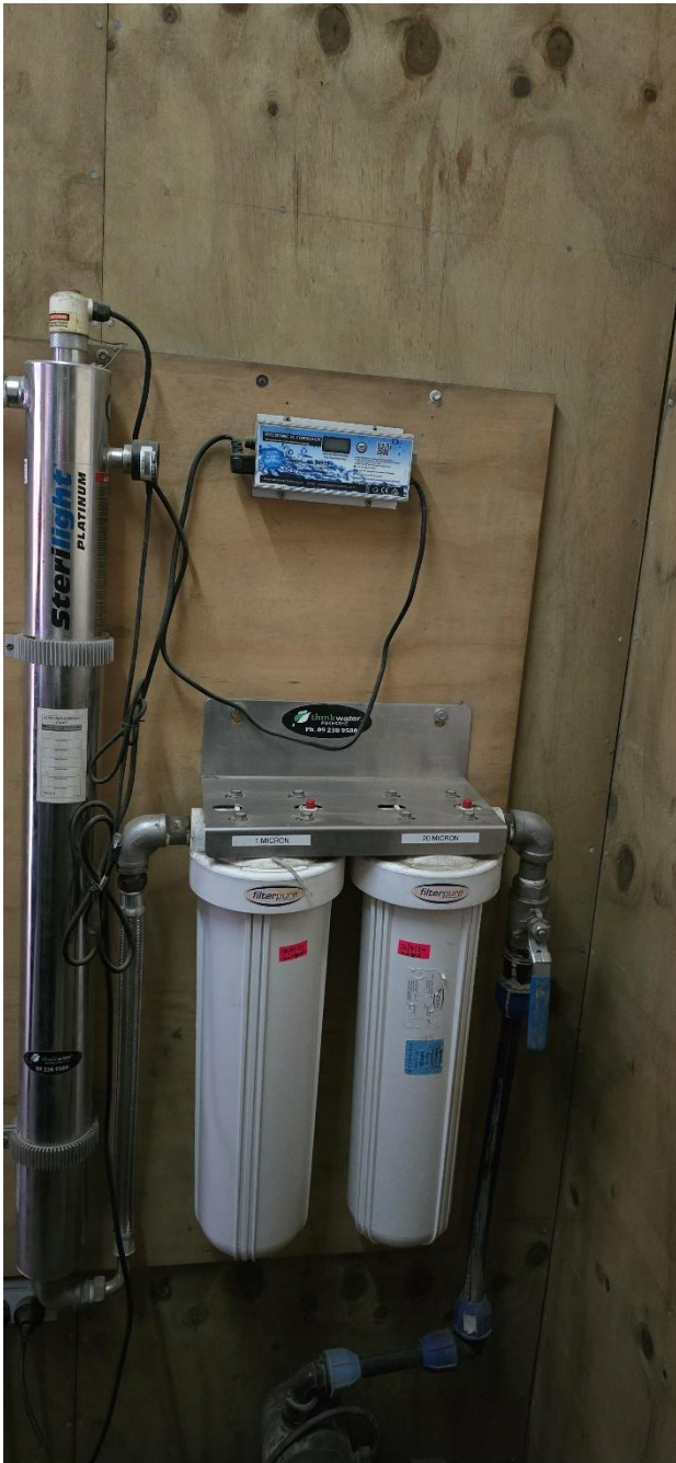
Figure 8: Water filtration system, internally located within operating theatre building.
