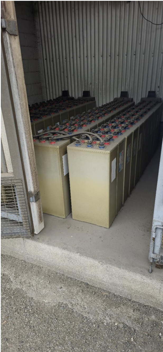
Figure 7: Battery storage, approximately 30cm above ground level.
