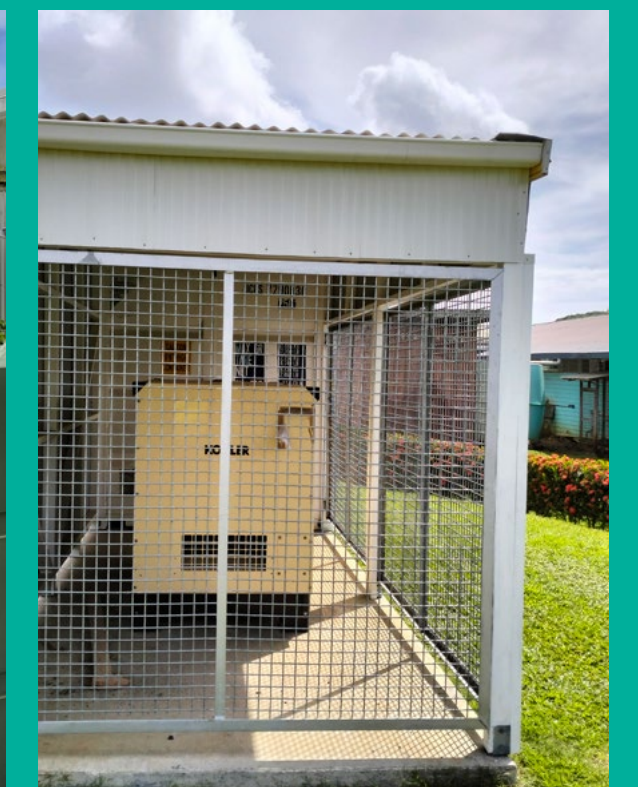
Papua New Guinea: Partial view of the 160-panel solar photovoltaic array at Madang Provincial Hospital Eye Clinic, delivering sustainable energy and ensuring reliable power supply.
